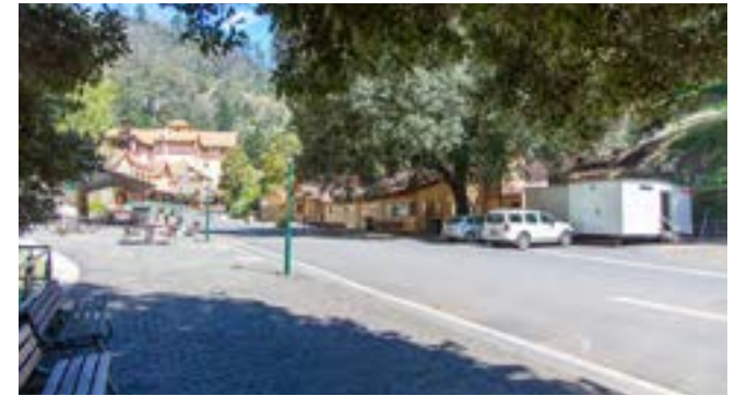
Jenolan Caves Road in the main visitor precinct
