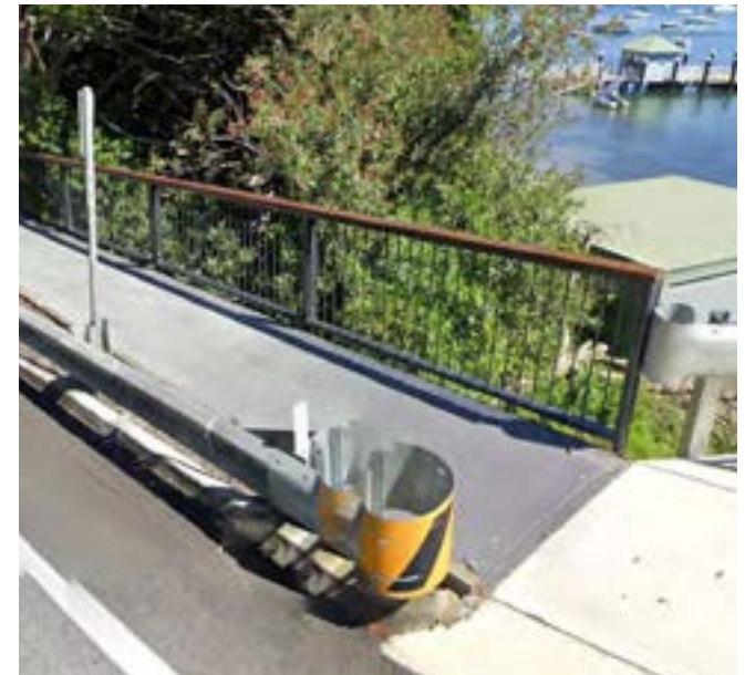
Suspended footpath along Barrenjoey Road, Palm Beach. Photo: Google Maps.
