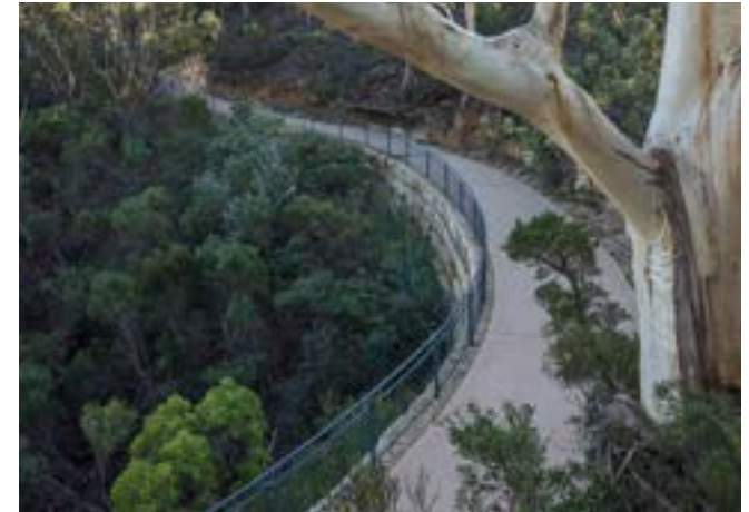
Concrete footpath with broom finish and warm tint. Location: Three Sisters Walk, Katoomba. Photo: NPWS.
