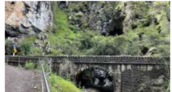
De Burghs Bridge
