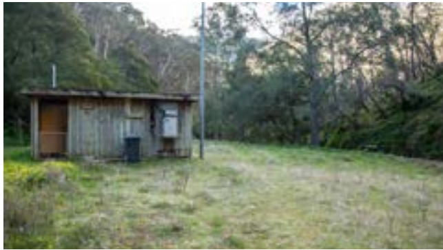
Disused toilet and shower facilities in the Campground and Utilities Precinct
