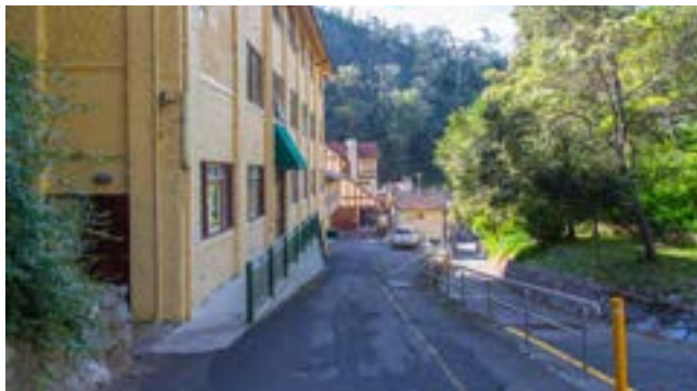
Entrance to Gatehouse Lodge
