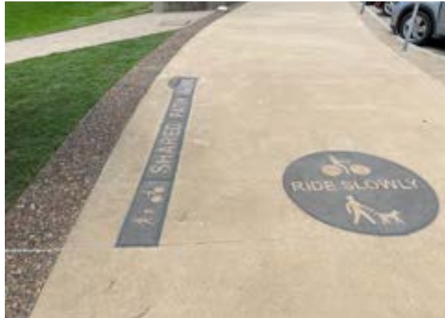
Exposed aggregate concrete footpath with integrated signage. Location: Bar Beach, Newcastle.
