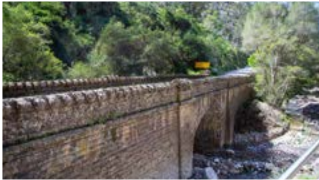
De Burghs Bridge, Jenolan Caves Road
