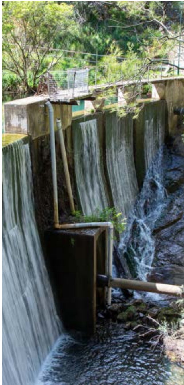
Blue Lake dam wall
