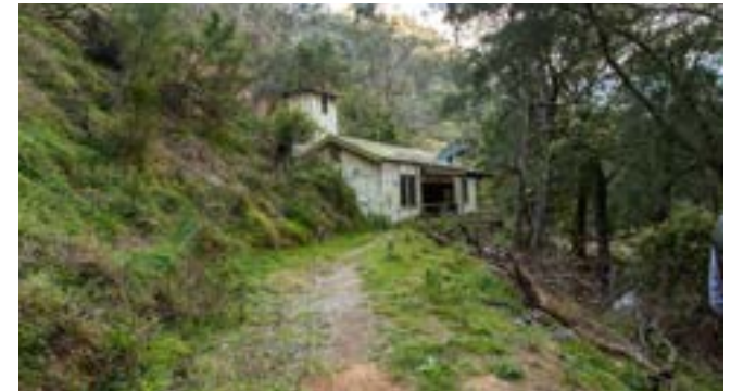
Old hydroelectric station
